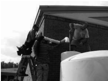
Fairview Cistern Install August 10, 2010
