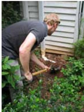
**STEP 2** - Pick a location close to your downspout and prepare a level area so that the barrel is stable (confirm using the level). Bricks or cinder blocks can be used to slightly elevate your barrel if needed.
