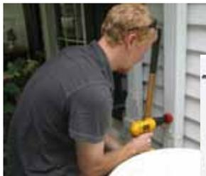
**STEP 4** - The kit comes complete with three hole saws that are the appropriate sizes to drill a downspout hole (2<sup>1</sup>/<sub>8</sub>inch), the connector hole (1<sup>1</sup>/<sub>2</sub>inch) and the spigot hole (1<sup>1</sup>/<sub>4</sub>inch). The largest hole saw (2<sup>1</sup>/<sub>8</sub>inch) is used to drill into the metal downspout. If you're cautious you can avoid pushing the drilled metal circle into the downspout.
