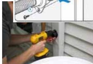
**STEP 5** - Now insert the FlexiFit Diverter which diverts a portion of the water from the downspout to the barrel but once the barrel is full allows rainwater to stay in the downspout. The cup is in my left hand. To insert the FlexiFit Diverter, simply pinch the cup upwards before inserting straight into the hole in the downspout (don't twist). Make sure the arrow on the front of the diverter is facing up. Attach the Diverter to the downspout using the two screws included with the Kit.
