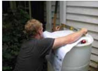
**STEP 3** - Next slide the level towards the downspout. The hole for the diverter will be drilled even with the height of the barrel. Don't drill too high or too low.
