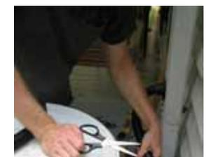
**STEP 9 & 10** - Simply screw the plastic spigot into the threaded rubber seal and put the barrel back into place and insure it's level. Insert the 3ft hose into the diverter and using the scissors cut off any 12 inch sections that are not needed to reach the barrel. Push hose into the connector seal in back of the barrel.
